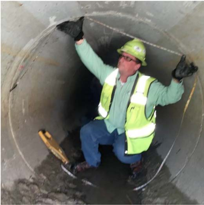
FIG. 1 Person Entry Inspection
